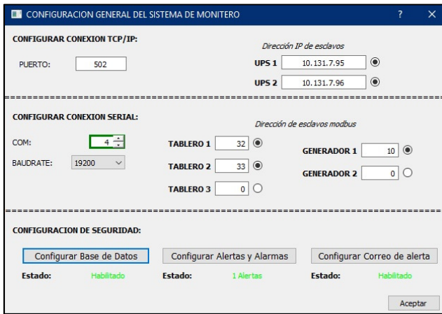
Fig. 17. Successful configuration of the power control and backup equipment of the ECU 911 Loja.
